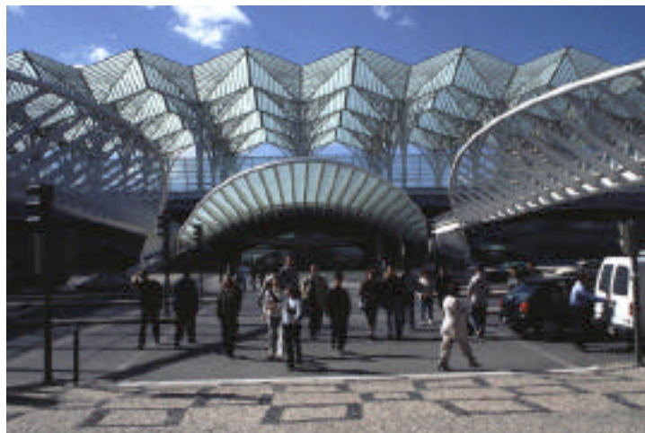
Lisbon Expo interchange station
