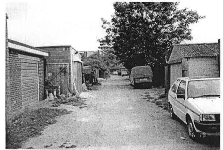
While the majority of backland areas are highly valued, the nature and character of backland areas does vary considerably
