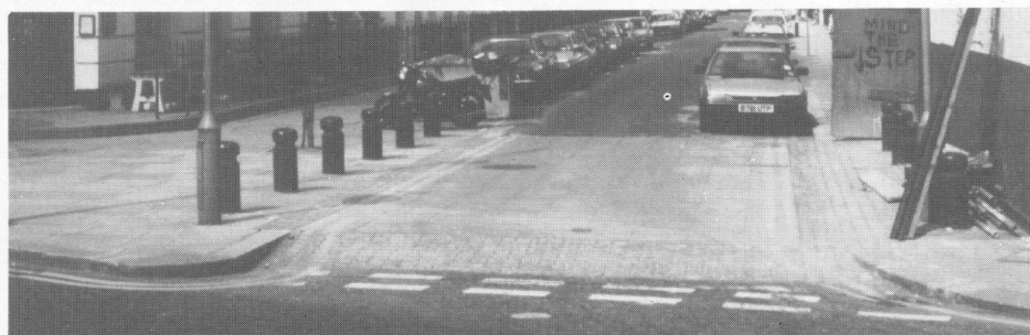
A raised carriageway provides a continuous footway across this T-junction at Millbank in Westminster, London.
