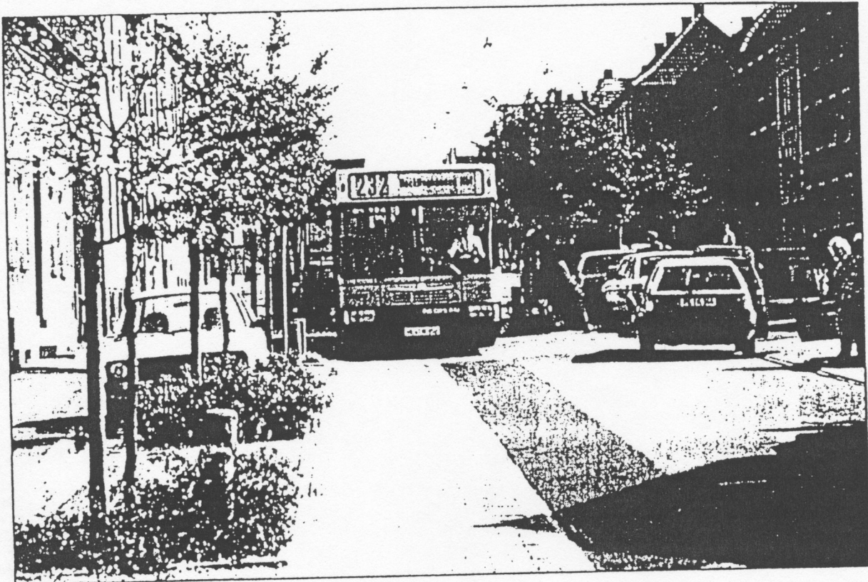
Combination Of Narrow Carriageway, Occasional Strips And A Bus Stop Located In A Single Lane
