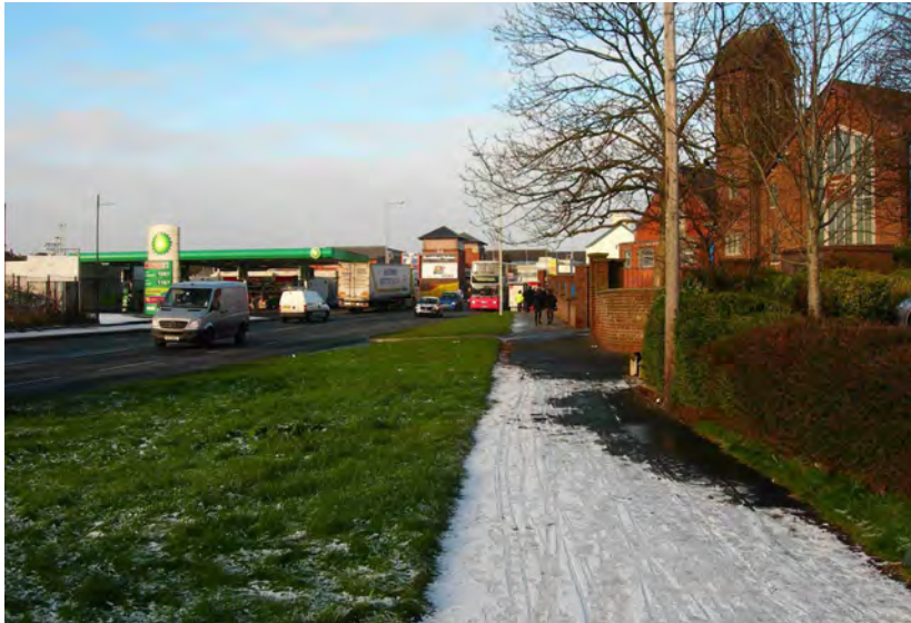
Figure 4.5: Good Quality Footway Outside Lidl
