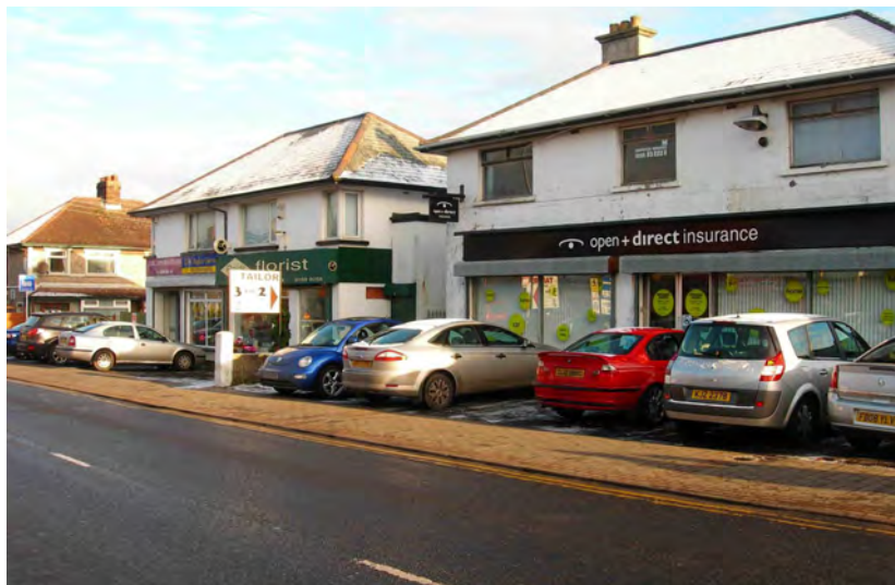
Figure 4.17: Forecourt perpendicular parking to A8
