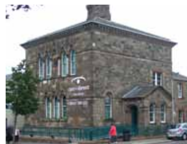
Use of local (Scrabo) stone for civic buildings
