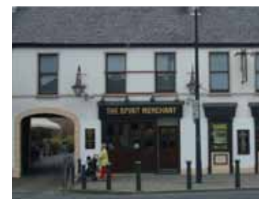
Arches providing access to rear yards
