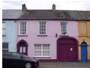
Coloured and painted render building frontages
