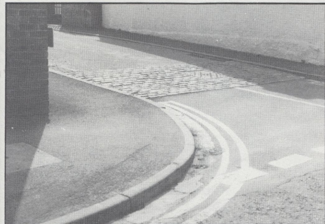
Cobbled surfaces can be dangerous to cyclists in the wet, particularly when they are cornering (Photograph: Cyclographic, from 'Cyclists and Traffic-calming')
