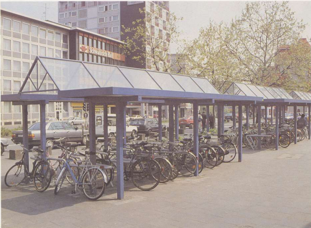
Cycle parking should be attractive and secure. Here covered cycle racks are located to allow supervision. Main station, Cologne, Germany.
