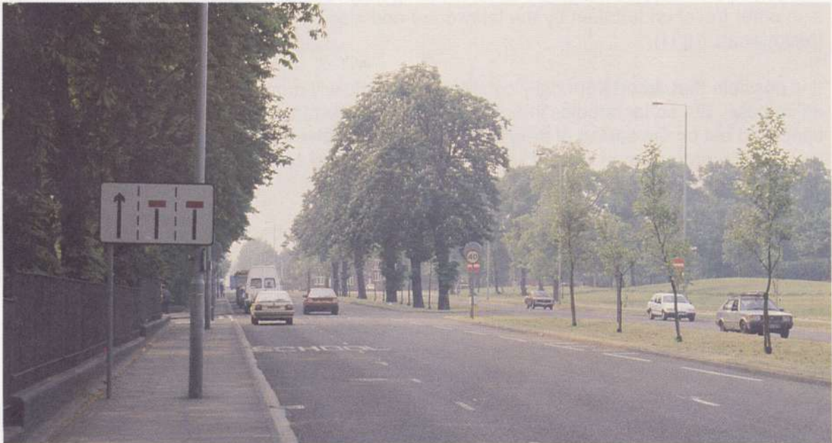
Past mistakes must end somewhere. Here a dual three-lane carriageway built in the 1970s will not be continued. Wandsworth, London.
