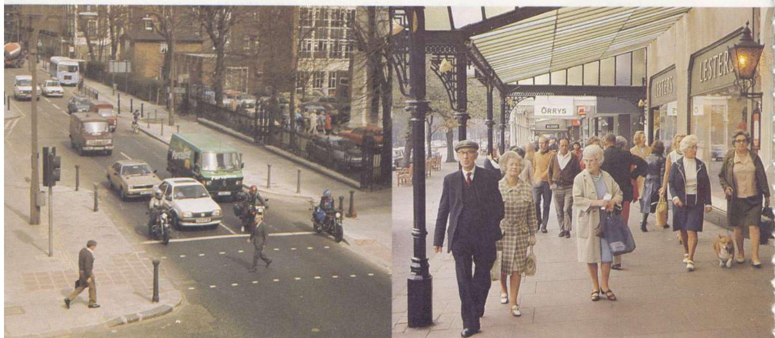
Reduction from four traffic lanes to two makes crossing easier. Tactile paving helps blind people to locate the crossing. Camden, London.
