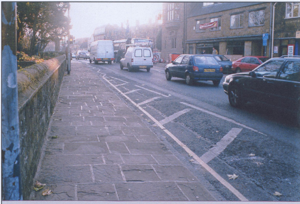
Heavy traffic like this could become more widespread throughout the day, and seven days a week, unless steps are taken to “cap” the growth of traffic in North Bar Street (pictured), Horse fair and South Bar Street. This is one of the most attractive parts of the centre of Banbury, and deserves to be less dominated by traffic.
