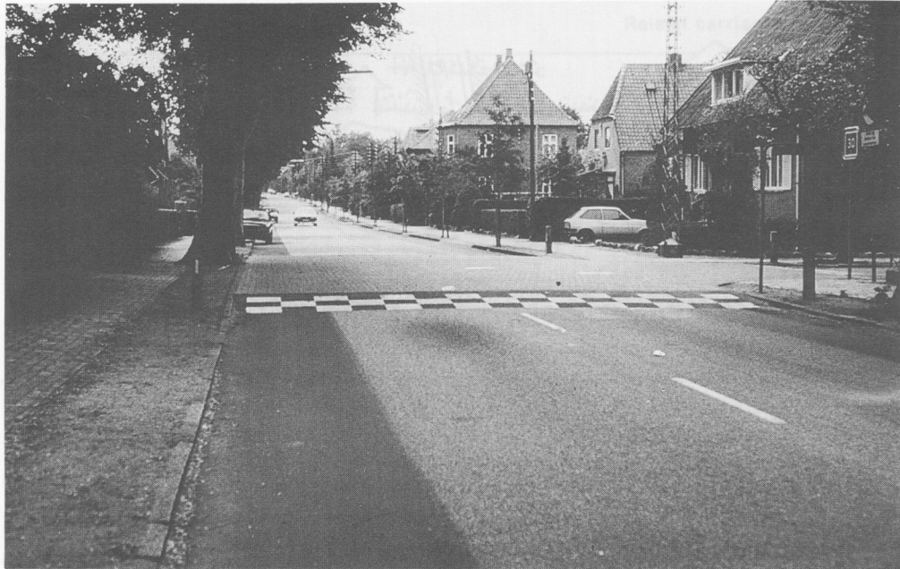
Fig. 10 Raised and ramped junction on a traffic road (50 kmph speed limit) in Odense, Denmark
