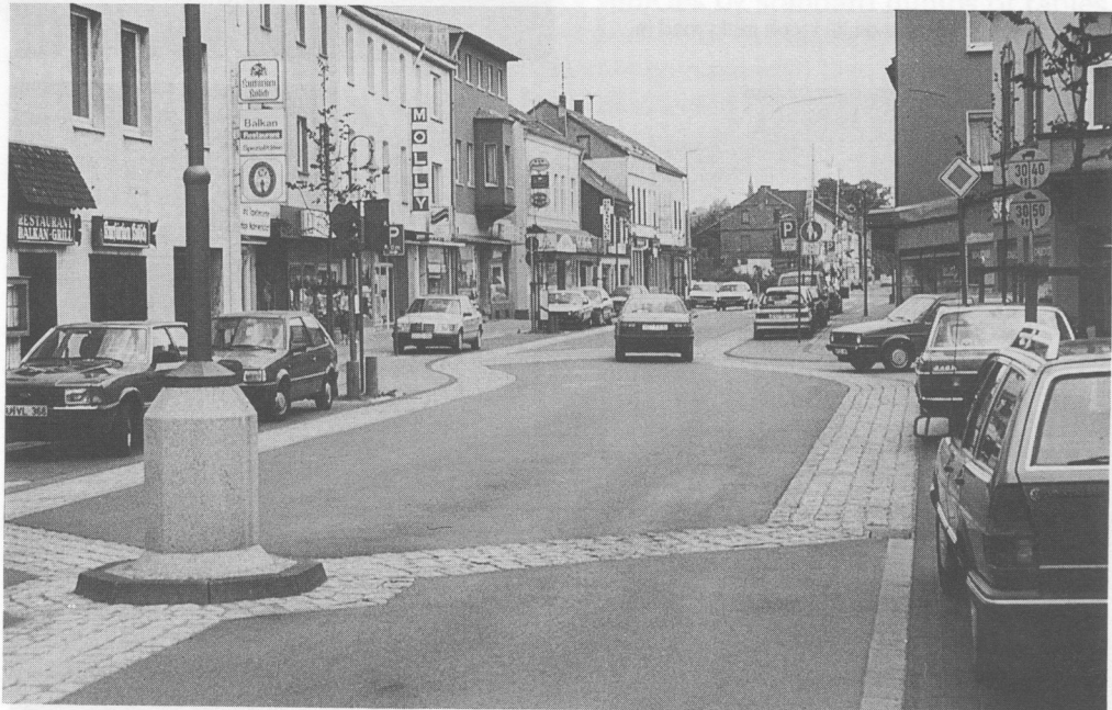
Fig. 14 Carriageways can be narrowed within multi-purpose strips (shown here at the side), which provide for large vehicles, parking manoeuvres, cyclists and pedestrians waiting to cross; Hennef, Germany
