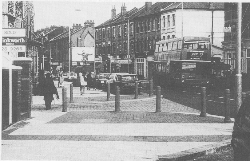
Fig. 9 St John's Hill in Wandsworth, London: a main road scheme with wide footways, sheltered parking and ramped side road entrances, similar to that shown in Figure 8
