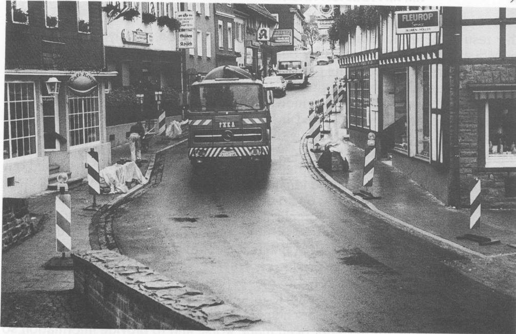
Fig. 15 Narrowing in progress on a Federal through road: lorries must pass single file between 4.5 metre width constraints; village centre, Much, Germany
