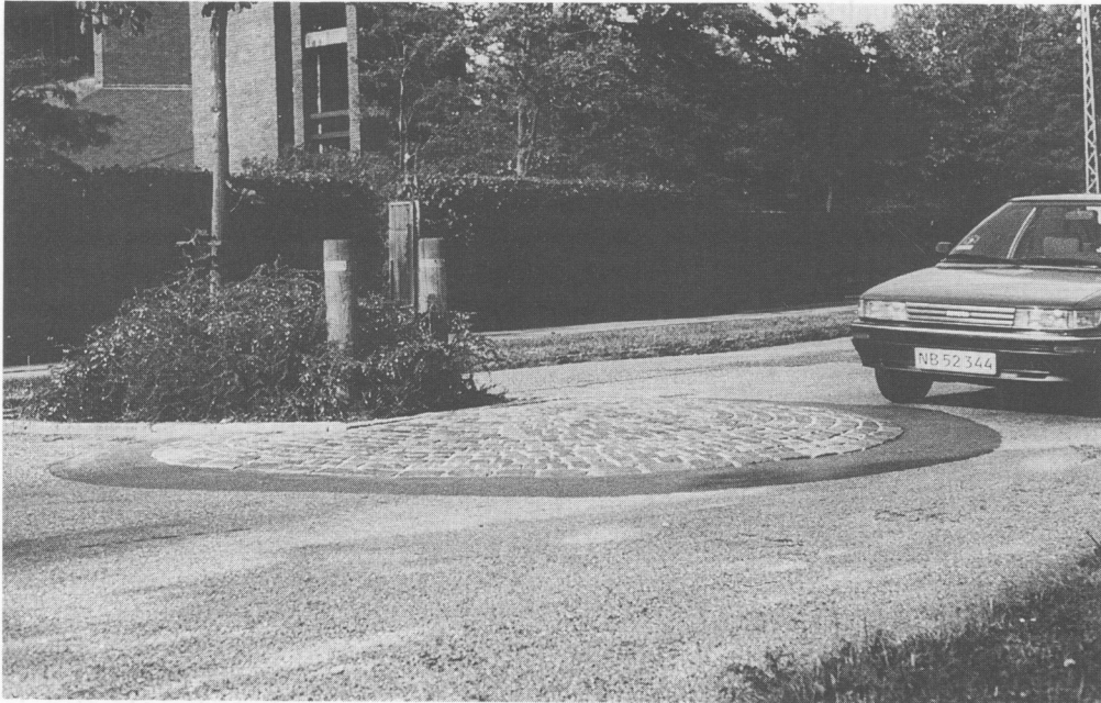
Fig. 16 Combined hump/chicane feature, used on wide 'school street' (30 kmph speed limit), Copenhagen
