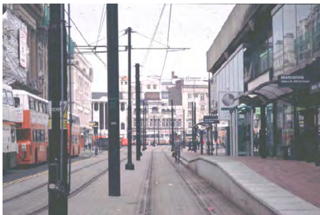
Unsightly infrastructure in Manchester city centre. Photo: Tim Pharoah.
