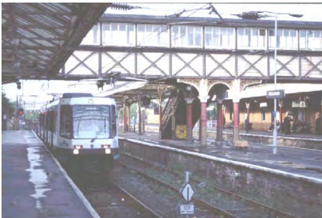
Former heavy rail station at Altrincham. Photo: Tim Pharoah.
