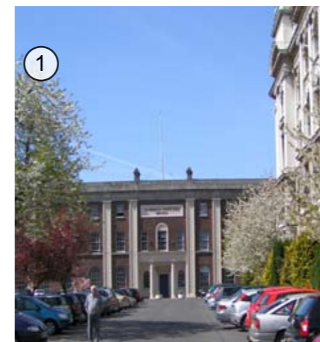
The grand 1810 facade of the Royal Belfast Academical Institution in College Square terminates the western end of the city's principal axis.
