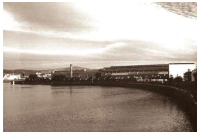
East Bank prior to demolition of the Sirocco Works
