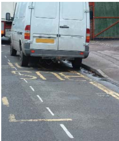
Confused markings for a bus stop bay.
