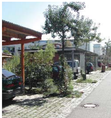
Integrated residential parking, Freiburg.
