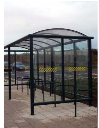
Cycle shelter and lockers Aberdeen.
