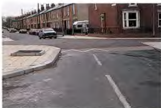
32: Junction treatment nearing completion in Stage 1 showing ramped plateau with chevron markings, extended footway, defined parking and tree "pocket". (Photo: K. Platt)
