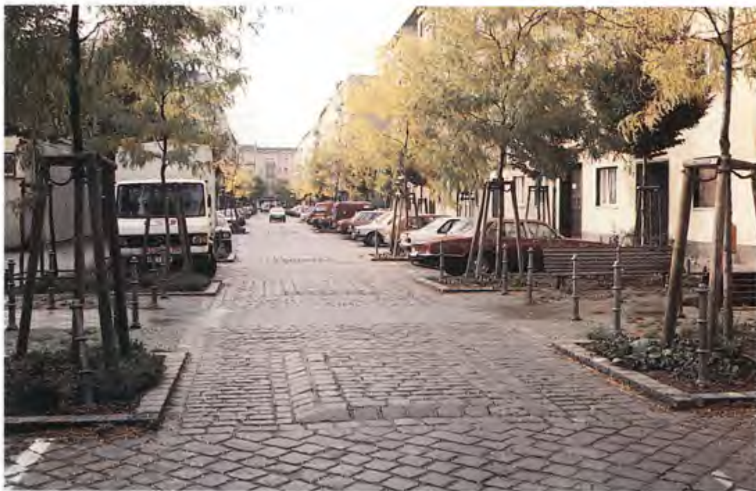
10: Speed reduction is achieved with the famous Berlin cushion, sometimes placed in twos or threes, as shown here. The optical width of the street is reduced with narrowings and intensive tree planting, which also helps to mask parked vehicles. (Photo: T. Pharoah)
