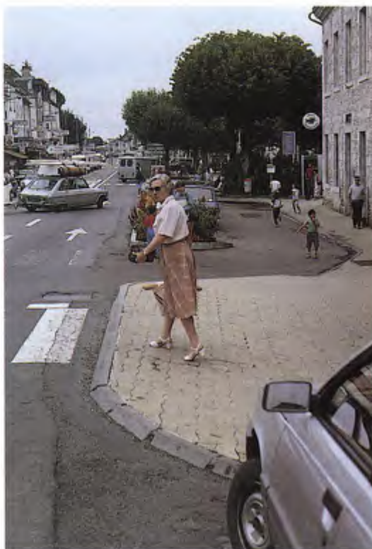
50: Footway extensions are particularly valuable at pedestrian crossings: they improve visibility and shorten the distance which pedestrians have to cross. Souillac, France. (Photo: T. Pharoah)
