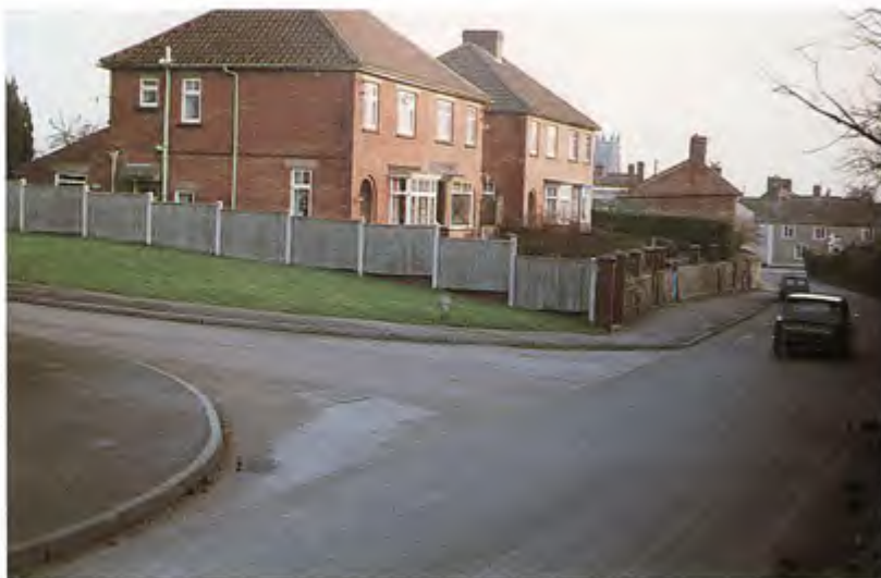
14: Excessive corner radii encourage speeding and are hazardous for pedestrians. (Photo: T. Pharoah)
