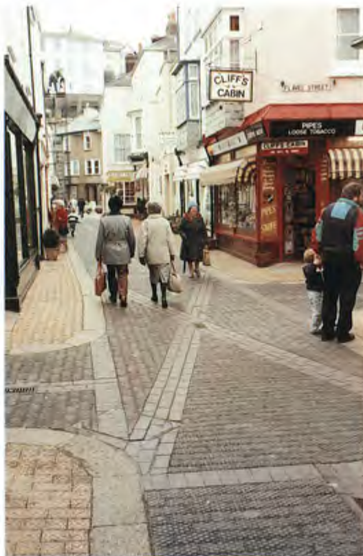
76: The carriageway and footway paved at one level. Traffic is calmed by the overall impression given by the layout of this street. (Photo: Devon County Council)
