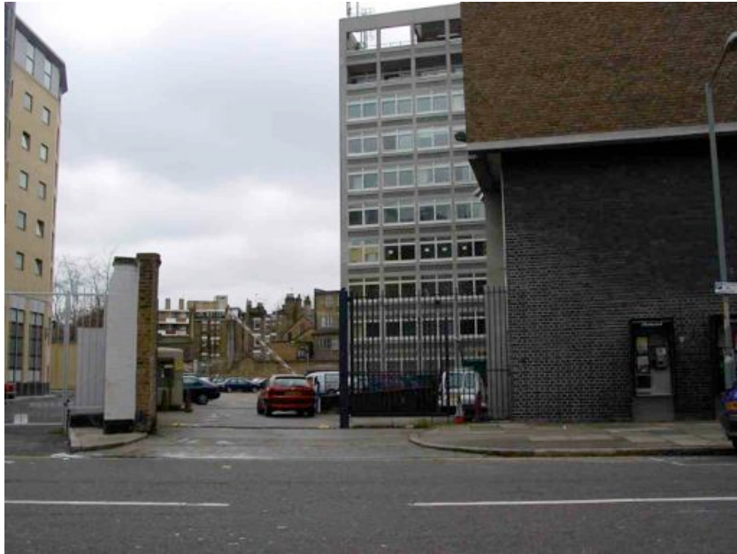
Friars House new Southwark JLE station, now fully refurbished for office use again. The car park and the student residence to the rear are visible on the left
