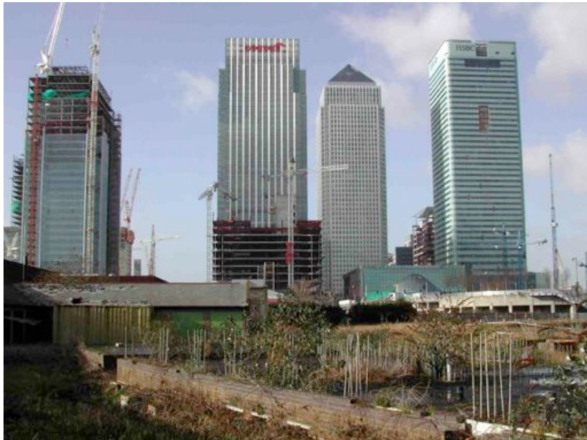
Wood Wharf site (foreground, showing proximity to existing Canary Wharf towers
