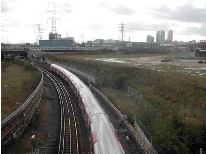
“Wrong side of the tracks!” The Channelsea site at West Ham. The station is at top left of the picture
