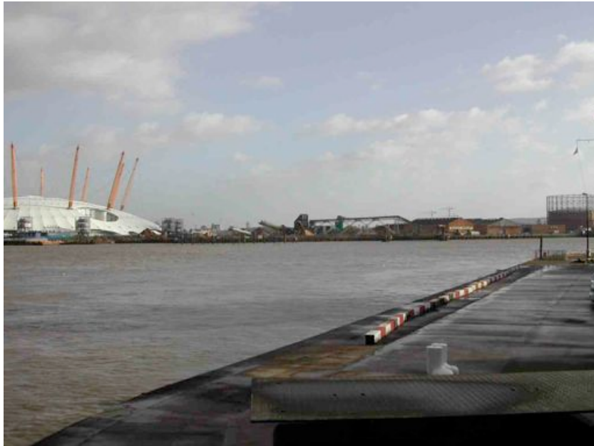
Delta Wharf to the right of the Millennium Dome: a major area for more intensive development
