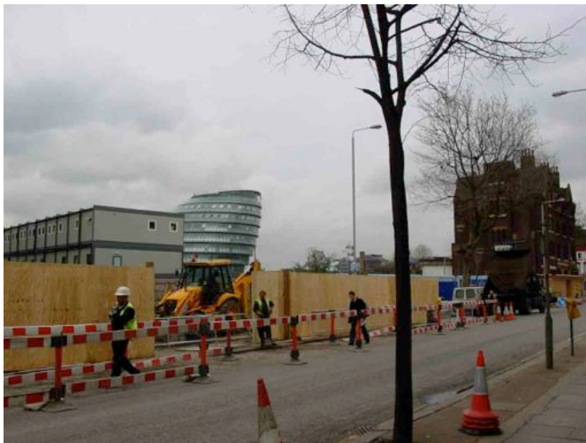
The new GLA rises above the rest of the “More London” major commercial development area (case study LB2)
