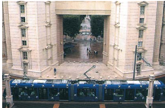
Montpellier(France): the tram stops directly outside the shopping centre
