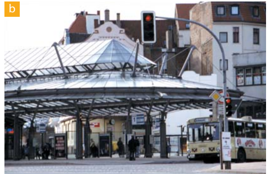
Lübeck: Good interchange between bus and rail
