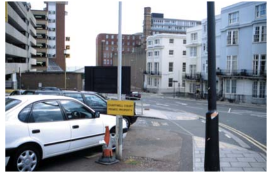
A private forecourt with vehicle access crossover creates an ill-defined route with unattractive walking environment
