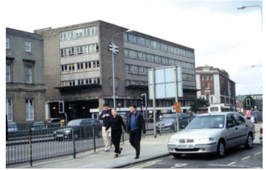
Welcome to the town: an unattractive station, and poor interface with the street
