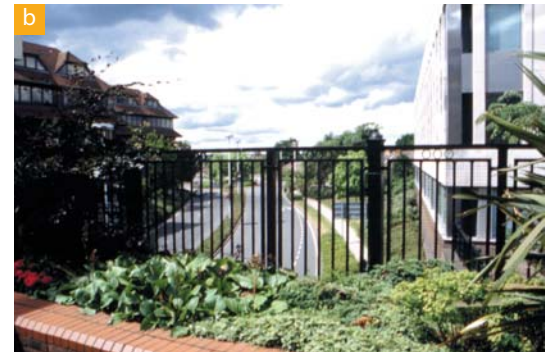
The view down to the dual carriageway: previously a severance problem. The bridge includes a substantial office building
