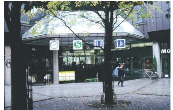
Stuttgart (Germany) has also brought direct rail access to the pedestrianised shopping centre, with underground stations for suburban trains and trams
