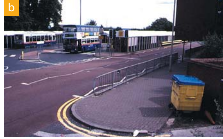
Bus station ripe for renovation.
