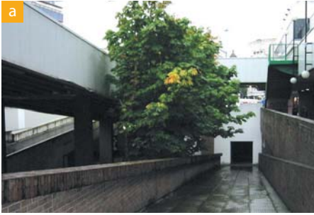
Poor pedestrian environment alongside city centre flyover
