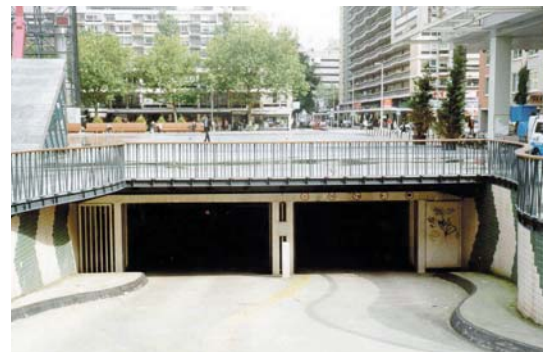
Car park provision under the city square in Rotterdam (Netherlands)
