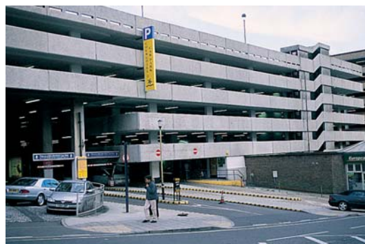
The pedestrian access to and from the multi-storey car park is not clear, and is dissected with car access ways and kerbs
