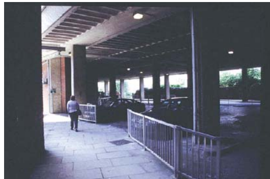
This car park exit has hidden corners and a poor layout
