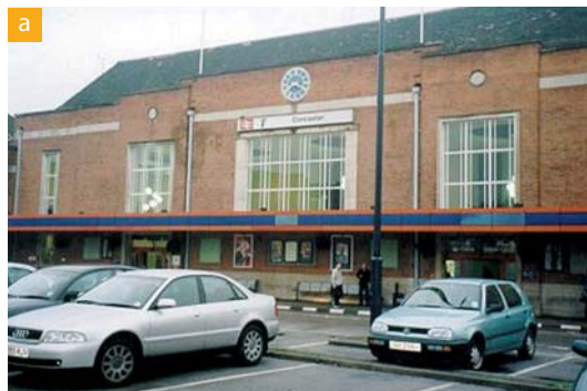
The station entrance
