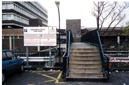
Bridge access from upper level parking
