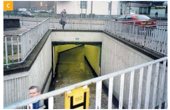
Pedestrians are routed through the subway - an unpleasant experience
