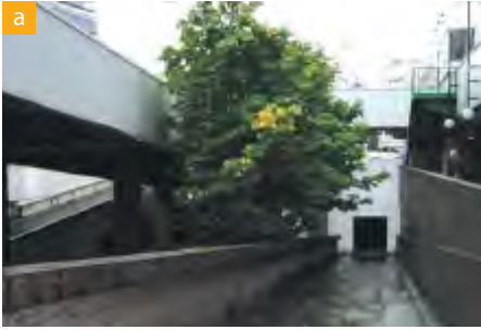
Poor pedestrian environment alongside city centre flyover
