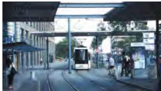
Bremen (Germany) airport tram stop linking to the city centre and main station
