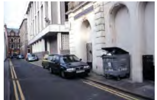
In this street, pedestrians are forced out by both waste storage and footway parking
