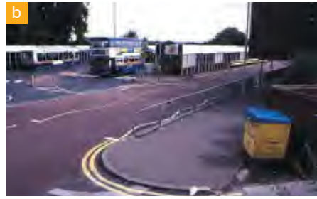
Bus station ripe for renovation.
