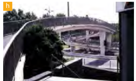
Bridge access to shopping mall (privately owned)
