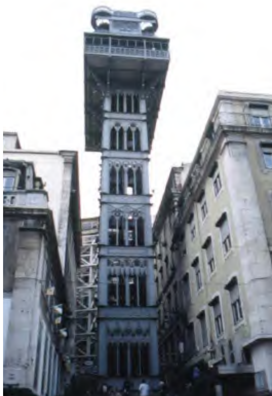
Sometimes dramatic changes of level call for dramatic solutions: a public lift in Lisbon, Portugal
