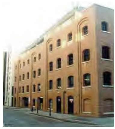
A well-planned car park at Bankside, London
