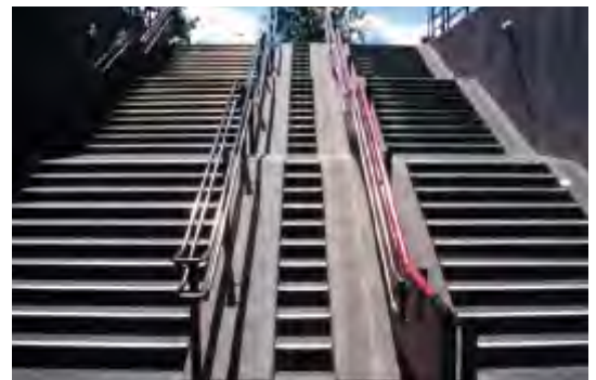
Ballerup (Denmark): central stairwell allows cycles, prams and wheelchairs up and down the level change
