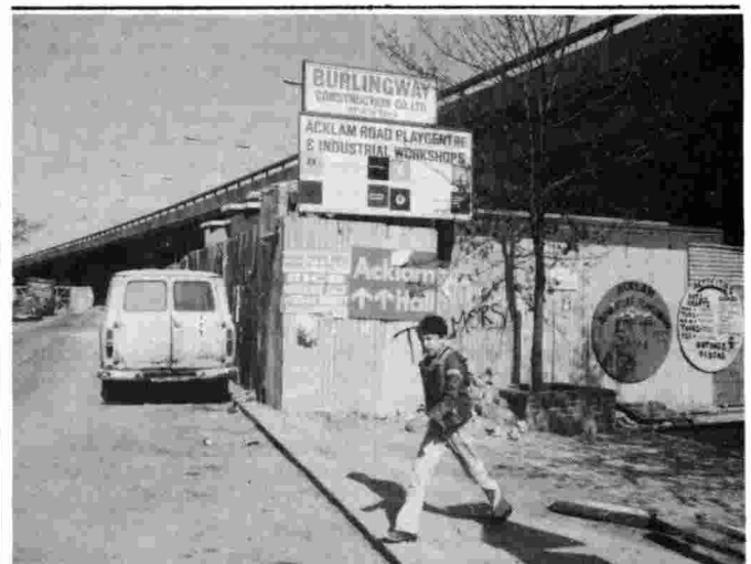
Twenty-four acres of land under the elevated section of the Westway in London have been taken over by the North Kensington Amenity Trust for community uses and industrial units. The trust is run jointly by local community groups and the council. Further details from Roger Matland, NKAT, 1 Thorpe Close, London W10 5XL. Tel: 01-969 7511.
