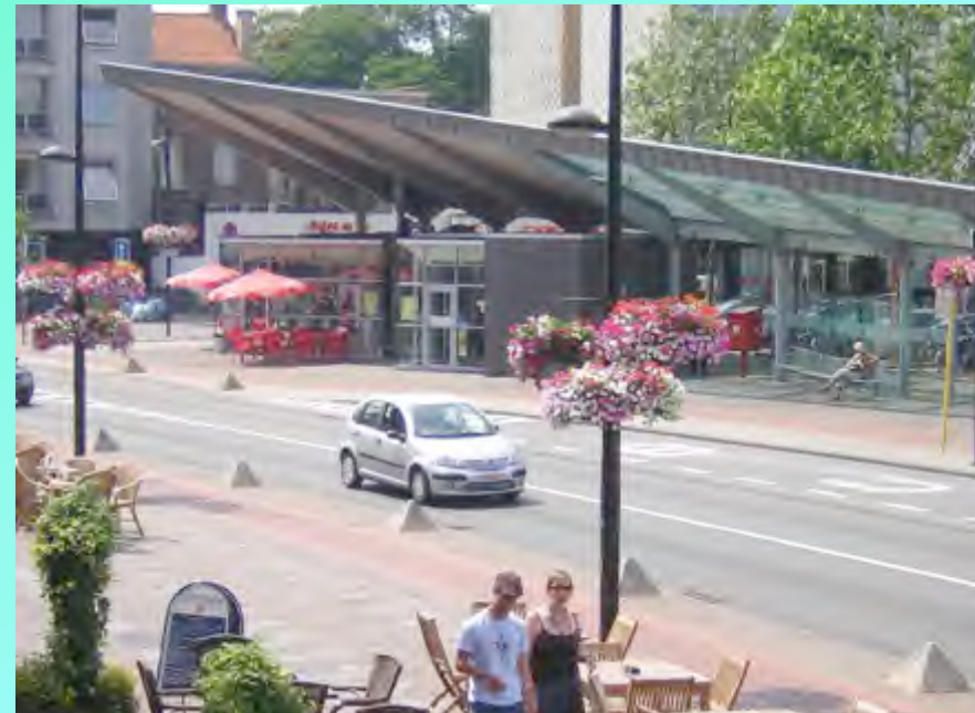
Landmark bus stop - Beveren, Belgium
