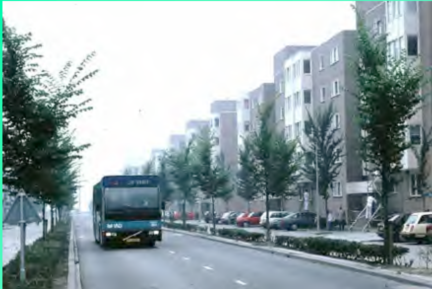
Busway through housing area
