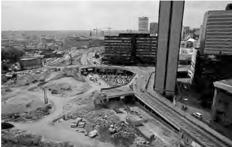
Above: Demolition of the ring road
