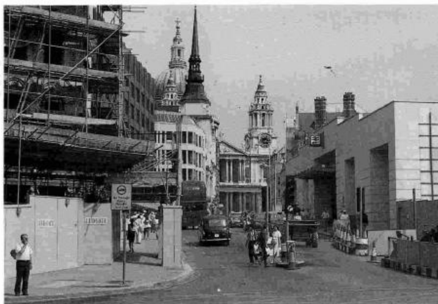
Figure 5. New offices and station near St Paul's, London.
