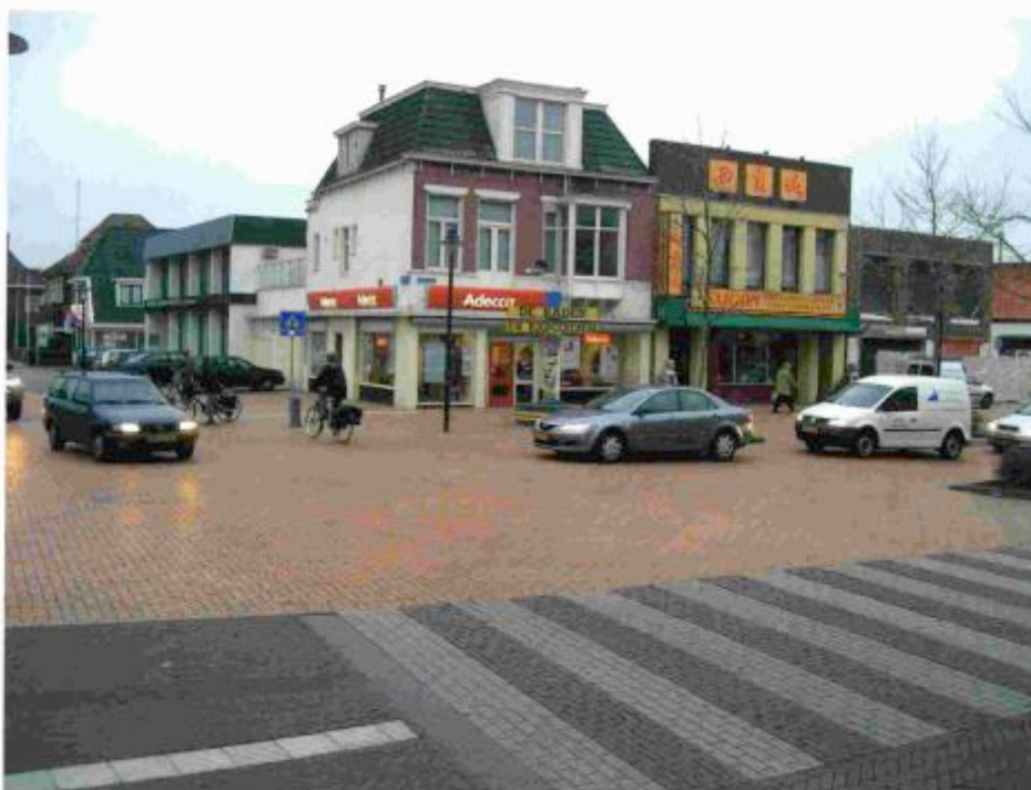
Shared space crossroads carrying over 20,000 vehicles per day at Drachten in the Netherlands – note quasi-zebra crossing with tactile approach
